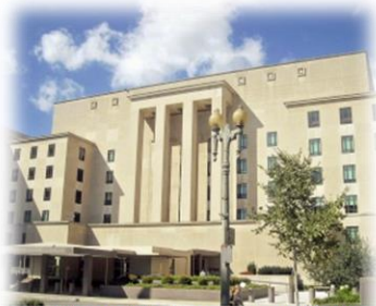
The 7th floor of the Harry S. Truman Building
